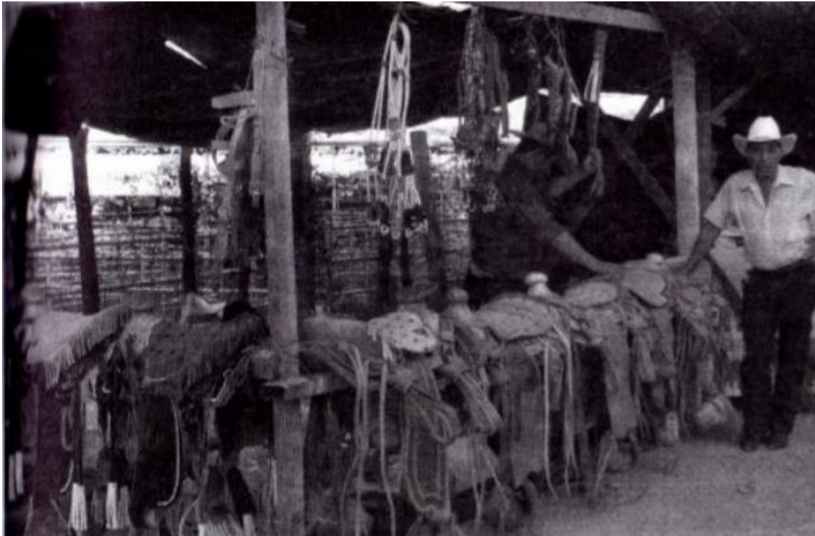
The making of each saddle combines leather and woodwork, the shaft is a single piece made of walnut or mango wood.
