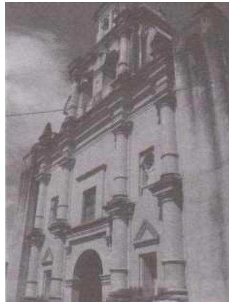
Santiago Jocotán. Chiquimula. Baroque: Movement of wall mass in columns. Suppression of the entablature between the first and second bodies.
