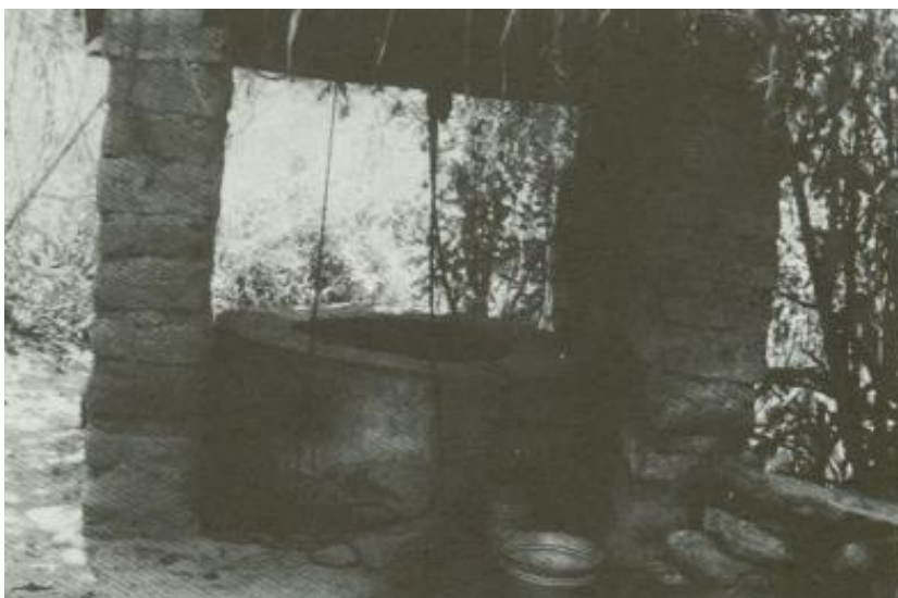
(d) ... a pulley, a tin can, the necessary cord, and a bucket to facilitate the transport of water.
