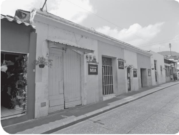
Image 12 Hurtarte House, traditional with parapet. (Chajón).
