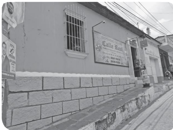
Image 18 Santos House, traditional with eaves and ashlars. (Chajón).
